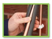
Without insulation, your house's hot-water pipes act as a gigantic radiator, transferring heat to the air so efficiently that any water in the pipes—even if it left the boiler at a toasty 105 degrees—is barely lukewarm 15 minutes later. So if you wash your hands to prep dinner then need to rinse a pot after you've finished eating, you'll have to wait for hot water all over again. The solution: Insulate pipes wherever you can reach them by encasing them in rubber or polyethylene foam tubes.
